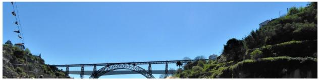
His second, and revered, Pont Dom Luis I, 1886, stretches Eiffel-tower-like 500' across the river. At the time it was the longest span of any metallic arch bridge in the world. Its two levels serve trains and (now) only pedestrians on the lower level. The bridge connects the funicular running along the remains of the Porto city wall across to upper and lower Gaia. The furthest downriver,
